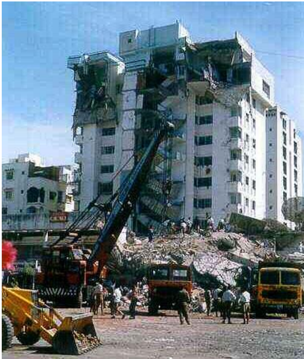
Collapse of a 11-story apartment building in Ahmedabad in 2001 earthquake
